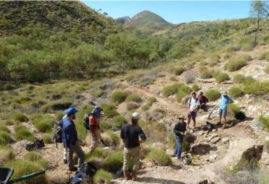
The FOLT walkers bumped into Snapper and his crew on their last walk (May 21-22) on Section 4 of the Trail, and were impressed to find the crew creating a zig zag into the trail (Rocky Cleft area). This small track re-alignment lessens the trail gradient and is sure to be welcomed by walkers with fully loaded packs.
